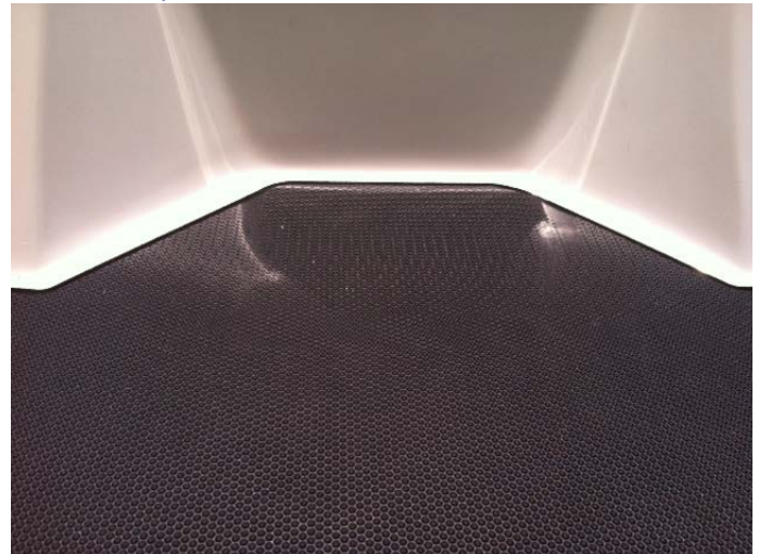
Concave areas of the gel-coat are where the occurrence is most likely.
